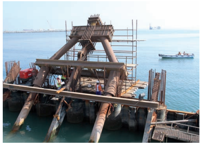
MV Pile test installation for 1,000-tonne tensile test.
