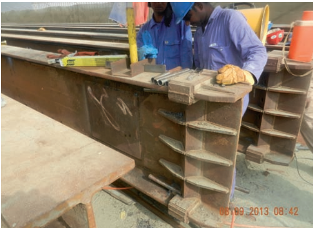
MV Pile head design.
